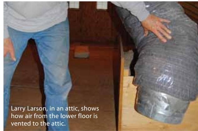
Larry Larson, in an attic, shows how air from the lower floor is vented to the attic.
