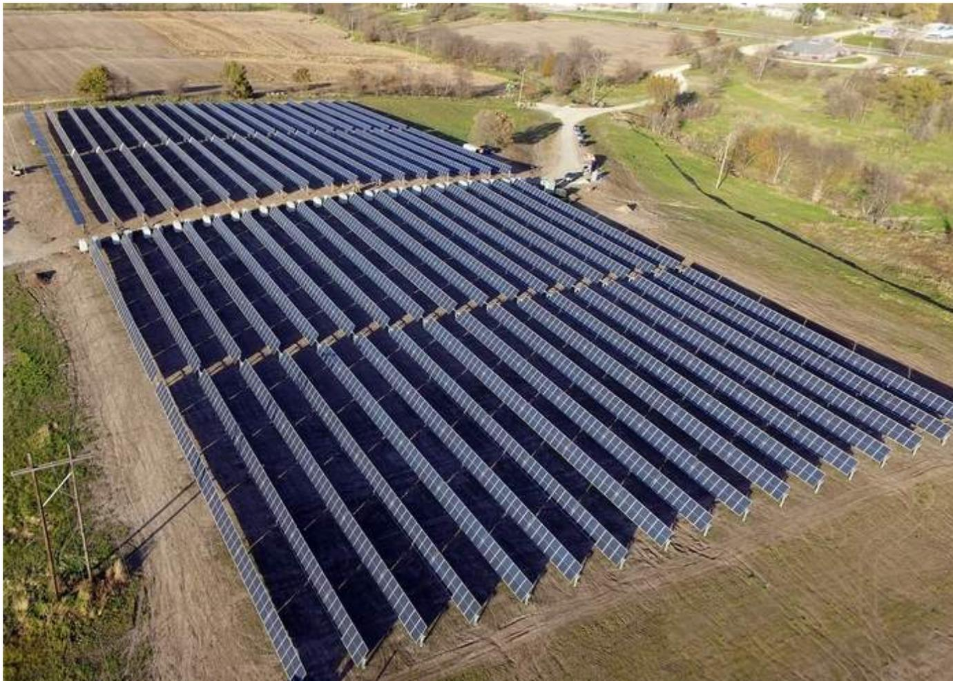
PHOTO COURTESY OF IDEAL ENERGY An aerial photograph shows the immense size of the 1.1 megawatt solar array recently built to power Maharishi University of Management. The array, and accompanying battery storage system, will provide one-third of the university's electrical needs.
